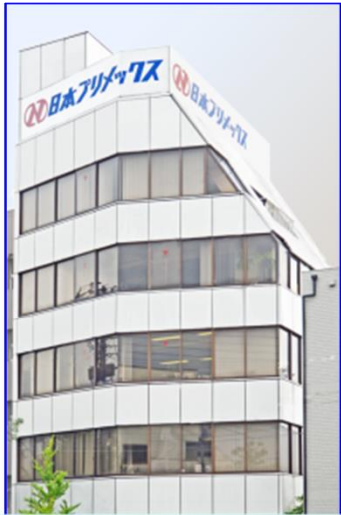
NIPPON PRIMEX INC. Headquarters in Tokyo
